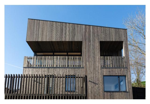
Larch that has been treated with a wood reactive agent that is non-toxic with a grey pigment. We apply this to timber decking and cladding in a factory-controlled environment. We recommend applying the SertiWOOD® Old Look on slow grown Larch that has been selected for its heartwood to ensure that a durable for use UC3 applications i.e. exterior above ground as not all larch is durable.
